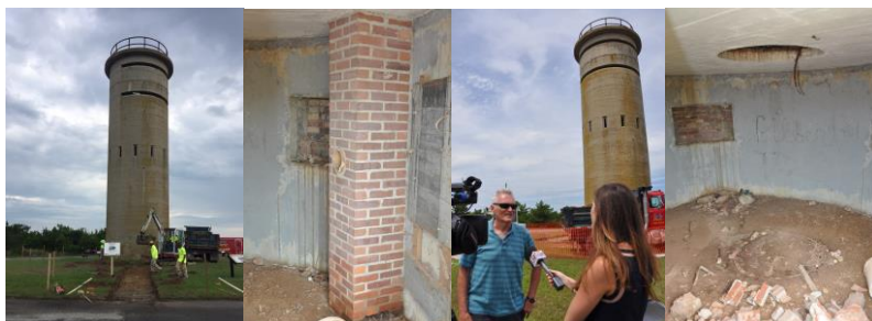
Restoration work continues on Tower #3; Larry Brown WBOC TV interview
